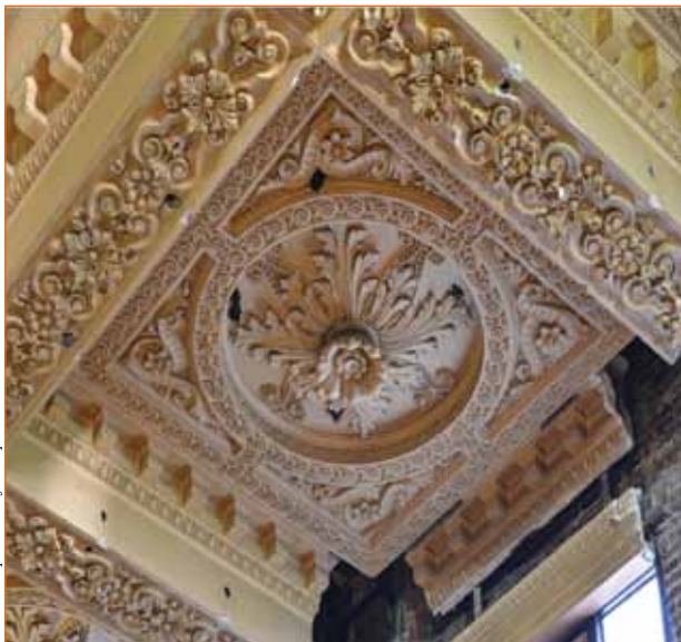
Rosette detail of King Street Station plaster ceiling
