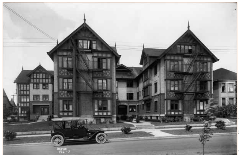
Historic view of Green Gables Apartments on 16th Ave. E.
