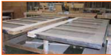
Wood door restoration at Washington Hall
