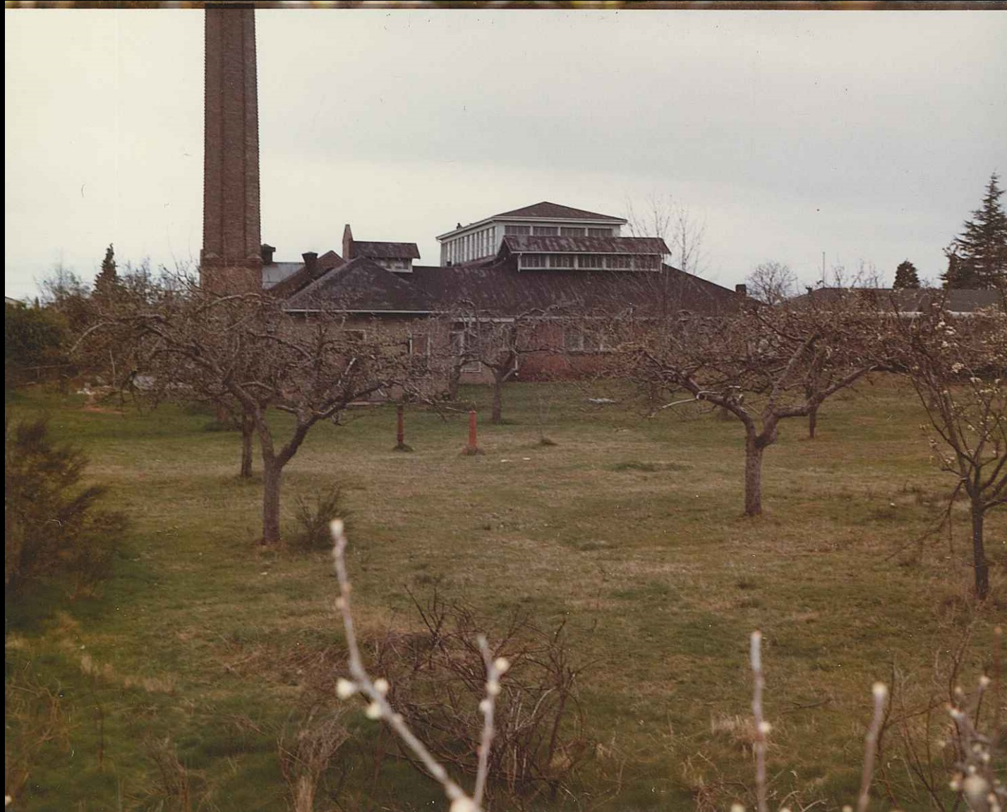
SE orchard with south annex 1975
