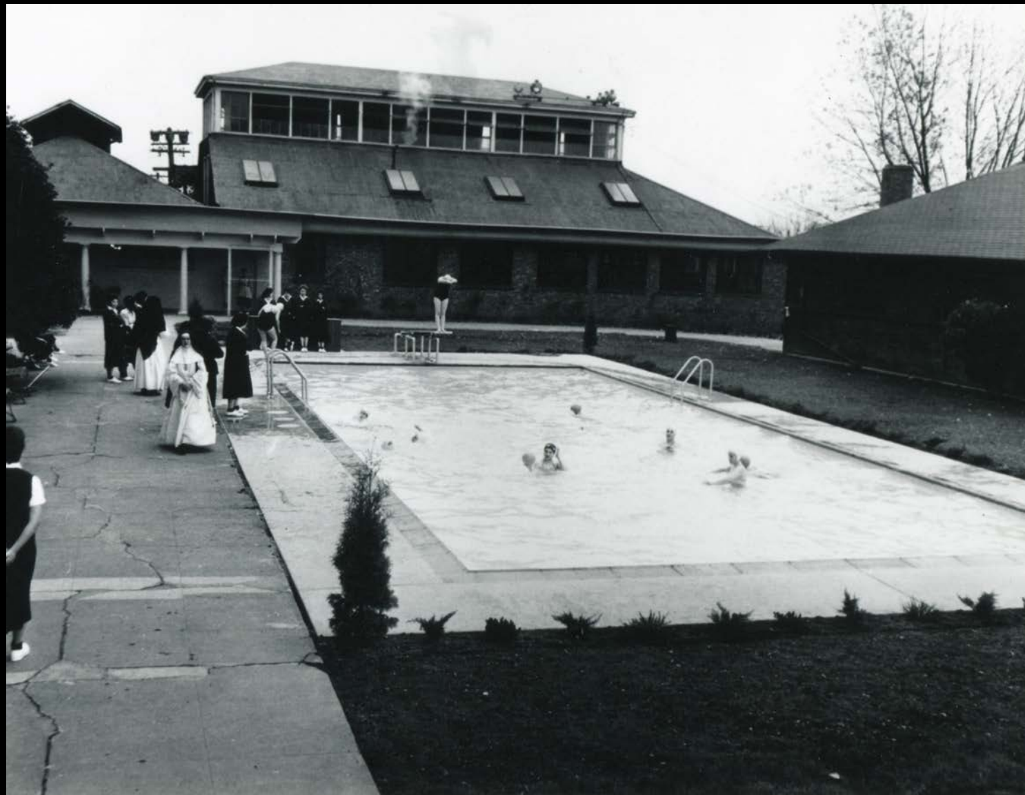
Pool, installed in 1959
