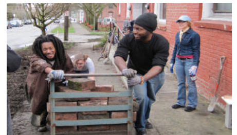
2010 The first phase of work begins.
