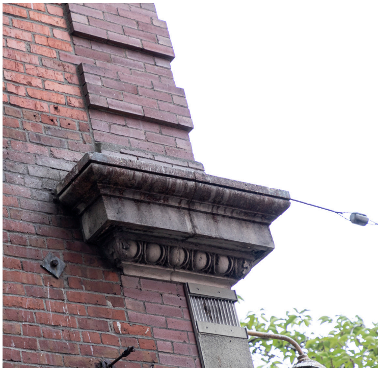
Figure 42. East facade belt course and brick veneer quoin detail.
