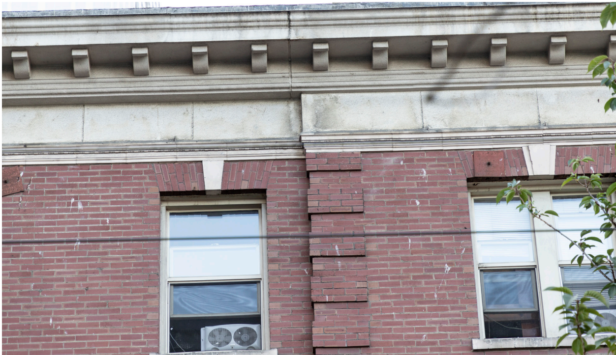
Figure 38. Upper north facade detail showing the cornice and brick detailing.
