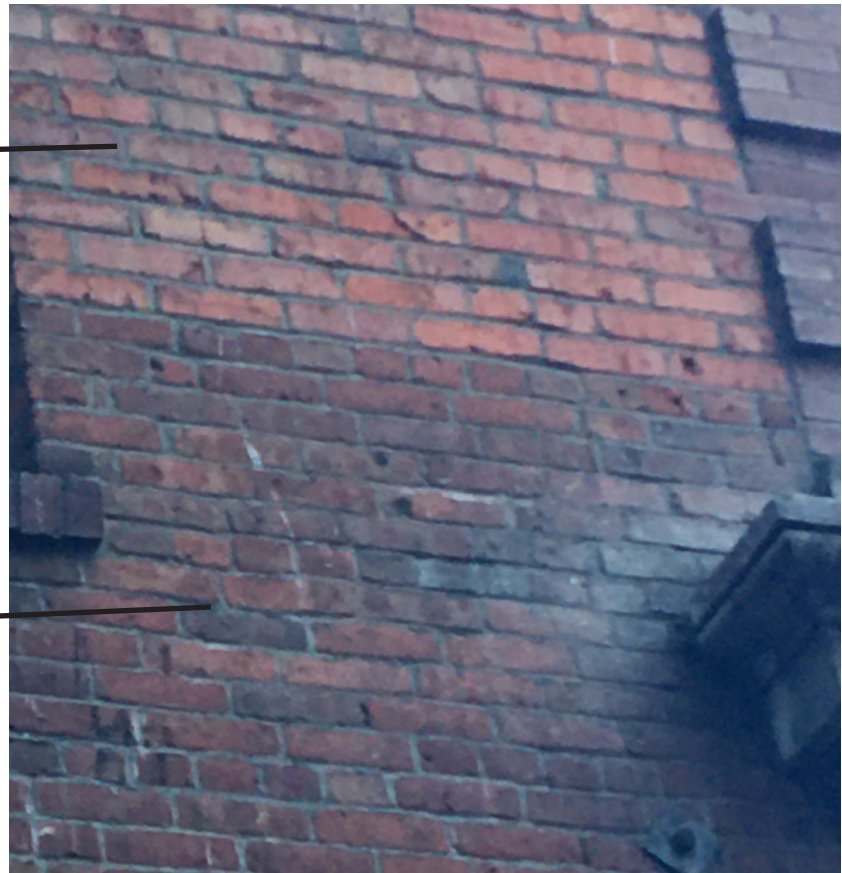
Figure 74. East facade showing the 1897 and 1908 brick transition at the second story. The 1897 brick extend the full length of the facade at the first story, with the 1908 brick at the upper two stories.
