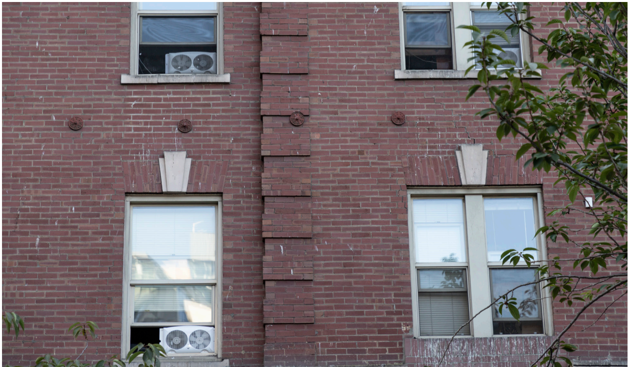
Figure 39. North facade upper story detail. The seismic ties stem from repairs after the 1965 earthquake.
