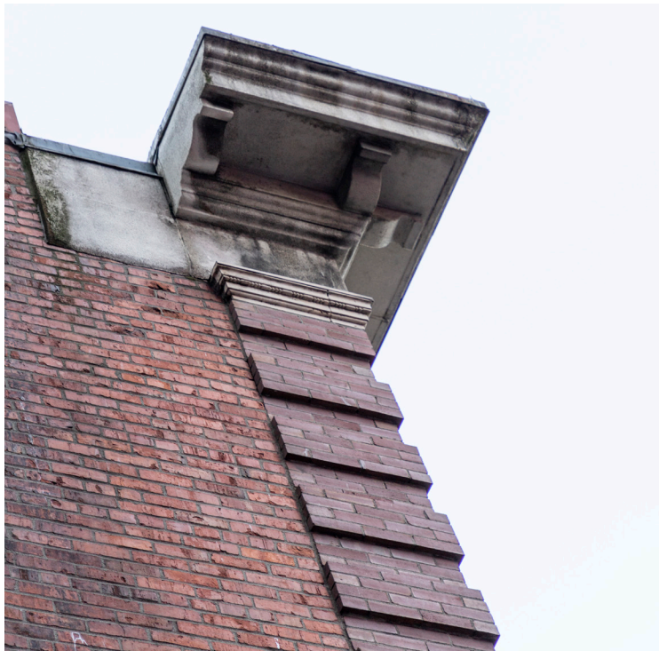
Figure 41. Cornice and brick veneer quoin detail.
