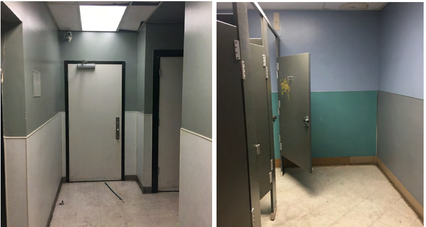
Figure 51. Service area, looking north within the northeast corner of this back of house area (above left), and a detail of the men's restrooms (above right) within the service area.
