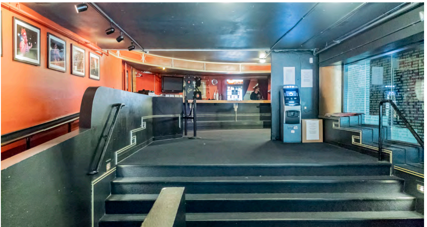
Figure 19. Showbox, entrance passageway showing the stairs, original south cheek wall and column, intermediate landing, and the original ticket window (originally a bar).
