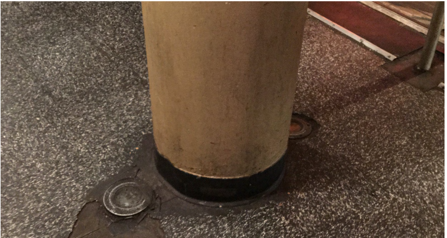
Figure 33. Showbox, detail of the floor lights original to the 1939 remodel that provided a light wash up the column.
