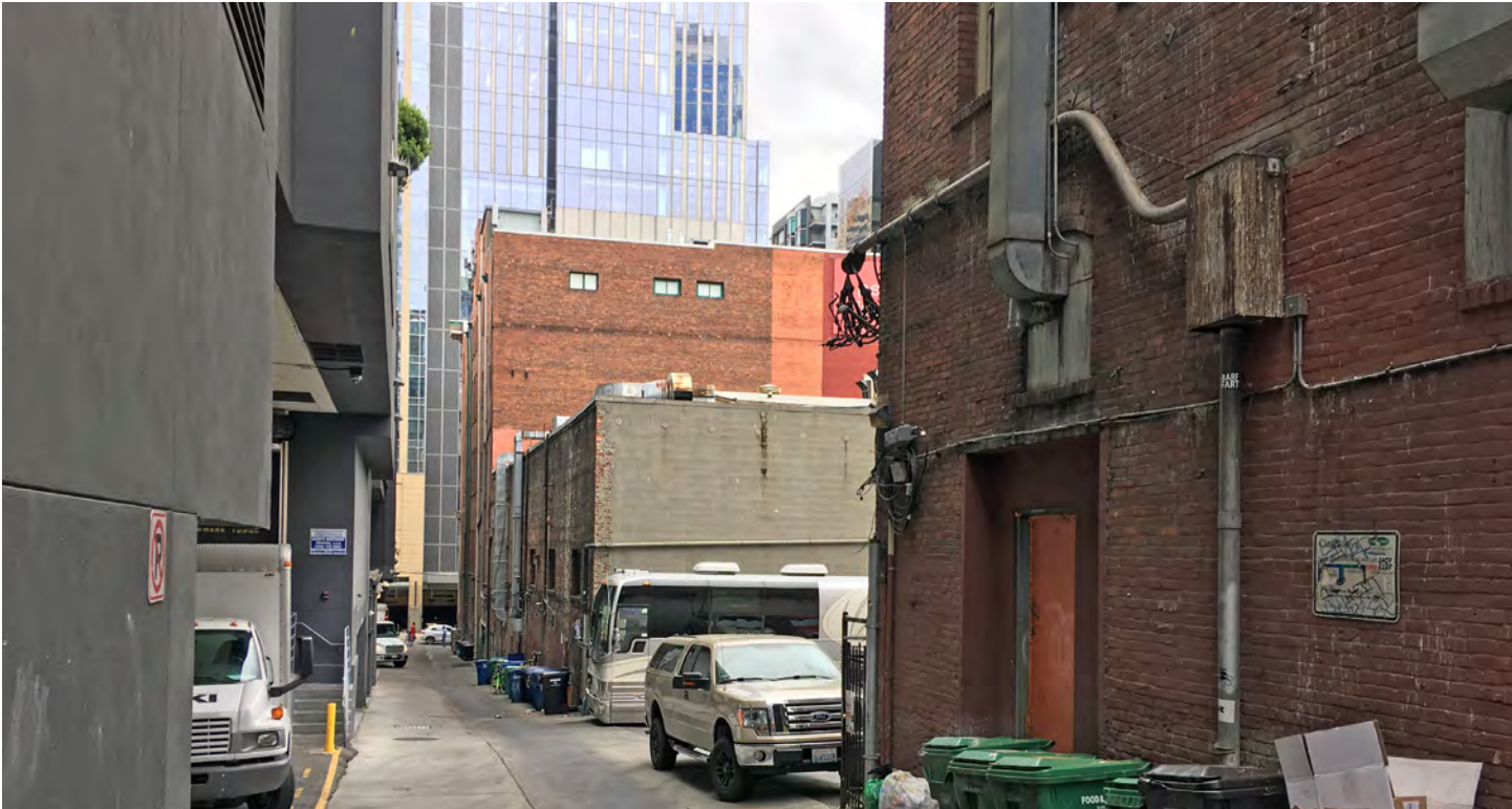
Figure 16. Context view, looking south along the alley that bisects the block. View from near Pike Street.
