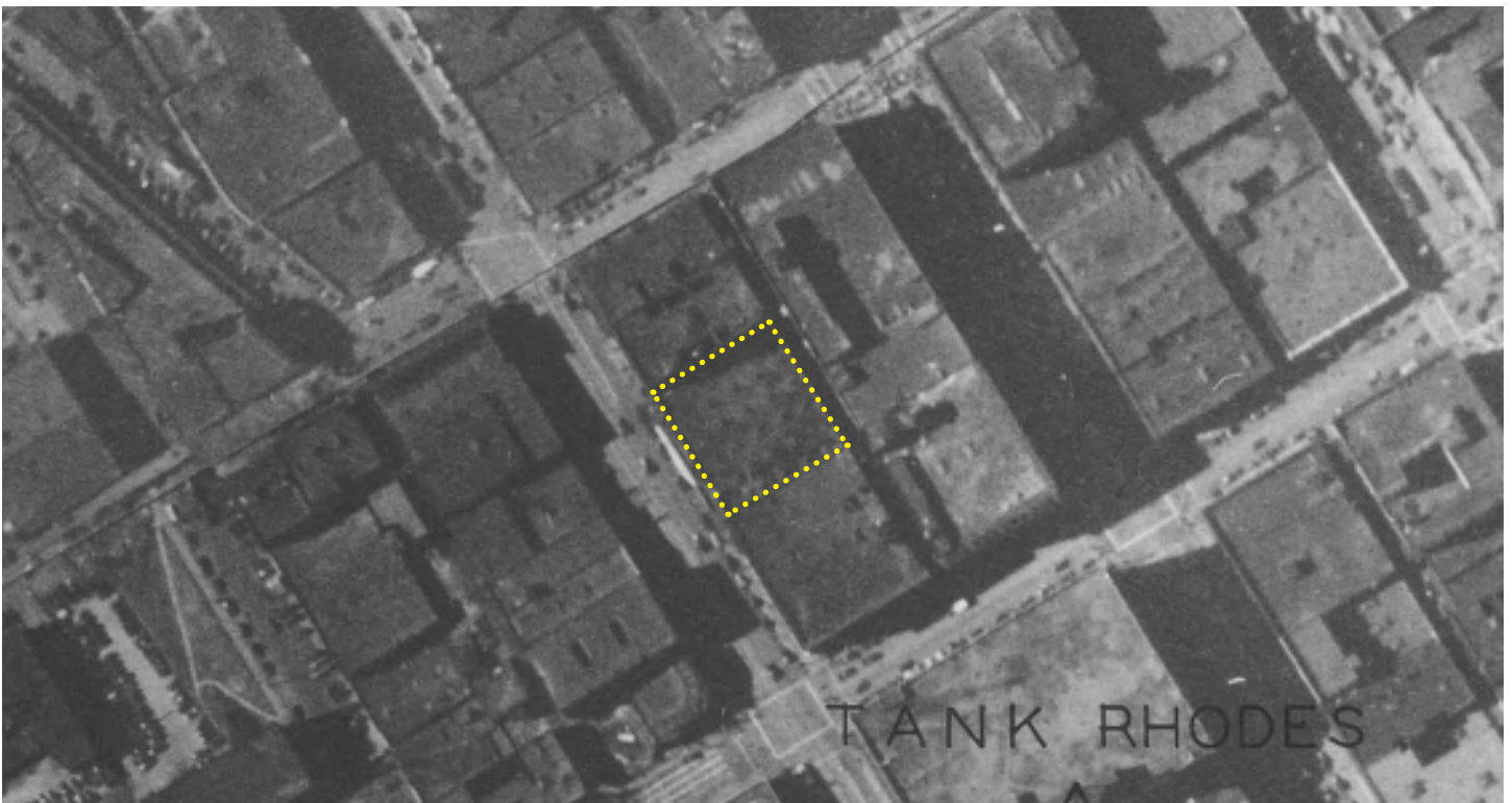
Figure 69. 1937 King County aerial showing the building (outlined in yellow dots) prior to the 1939 remodel. Note the elevated central truss roof portion for the vaulted ceiling at the second floor was part of the 1939 remodel.
