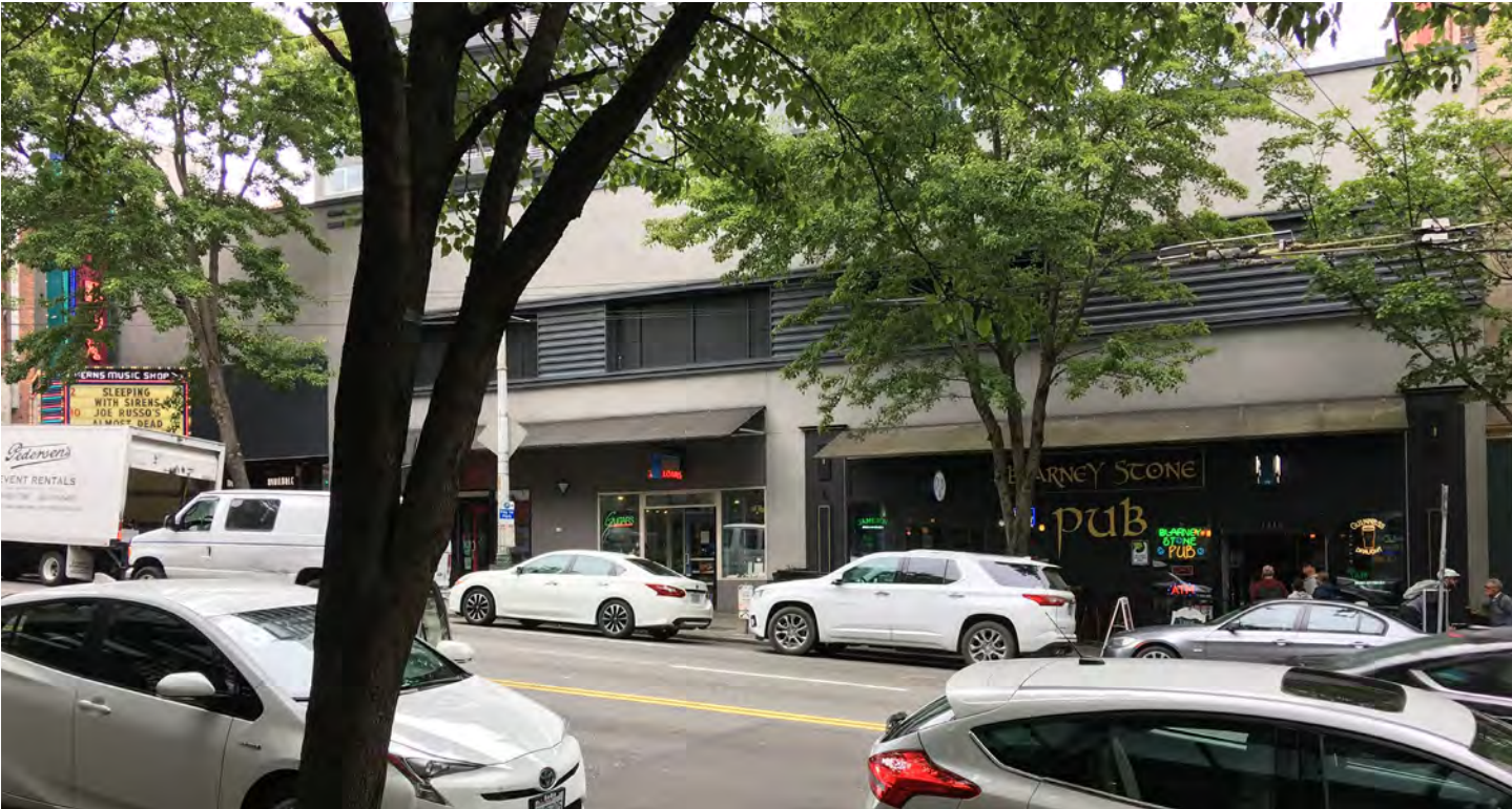
Figure 6. Front, west facade along 1st Avenue.
