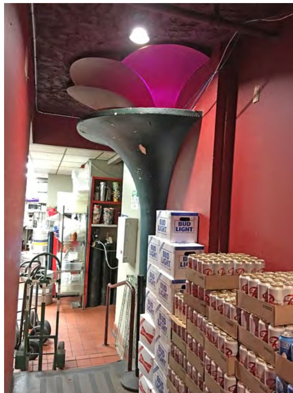
Figure 40. Showbox, detail of the walkway above the passageway from the west seating area into the kitchen. Note how later partitions were abutted up to the column elements leaving them intact.
