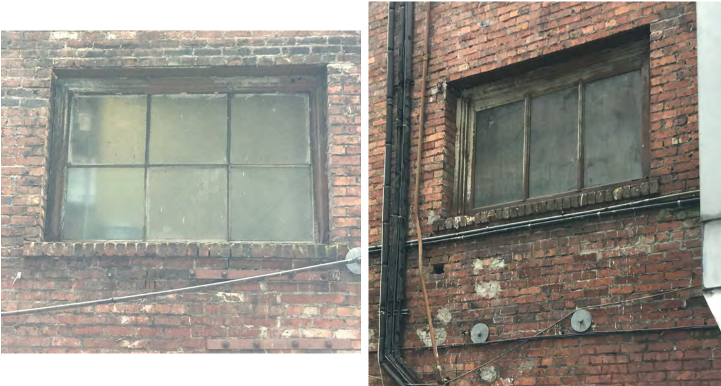
Figure 54. Alley facade, detail of the 6-lite (above left) and 3-lite (above right) sash along this facade.
