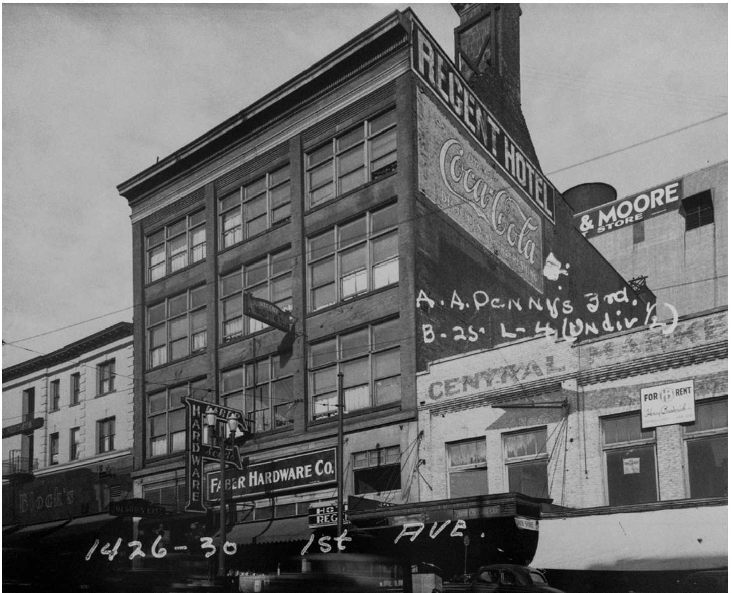
Figure 55. Ca. 1938 photograph showing the north portion of the west facade of the building when it was the Central Market, prior to the 1939 renovation that created the Showbox. This photograph also shows the Regent Hotel prior to its demolition and creation of the surface parking lot. Source: Puget Sound Regional Archives.
