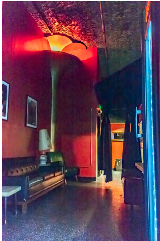
Figure 41. Showbox, outer green room looking south. Note how later partitions were abutted up to the column elements leaving them intact.
