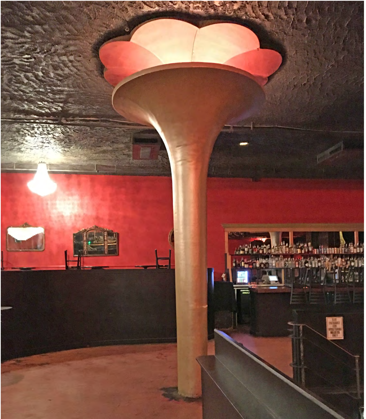
Figure 32. Showbox, detail of column original to the 1939 remodel. The core is a wood post with an outer plaster and wood form.
