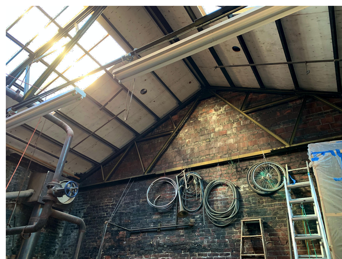
8 SOUTH ANNEX BOILER ROOM A702
