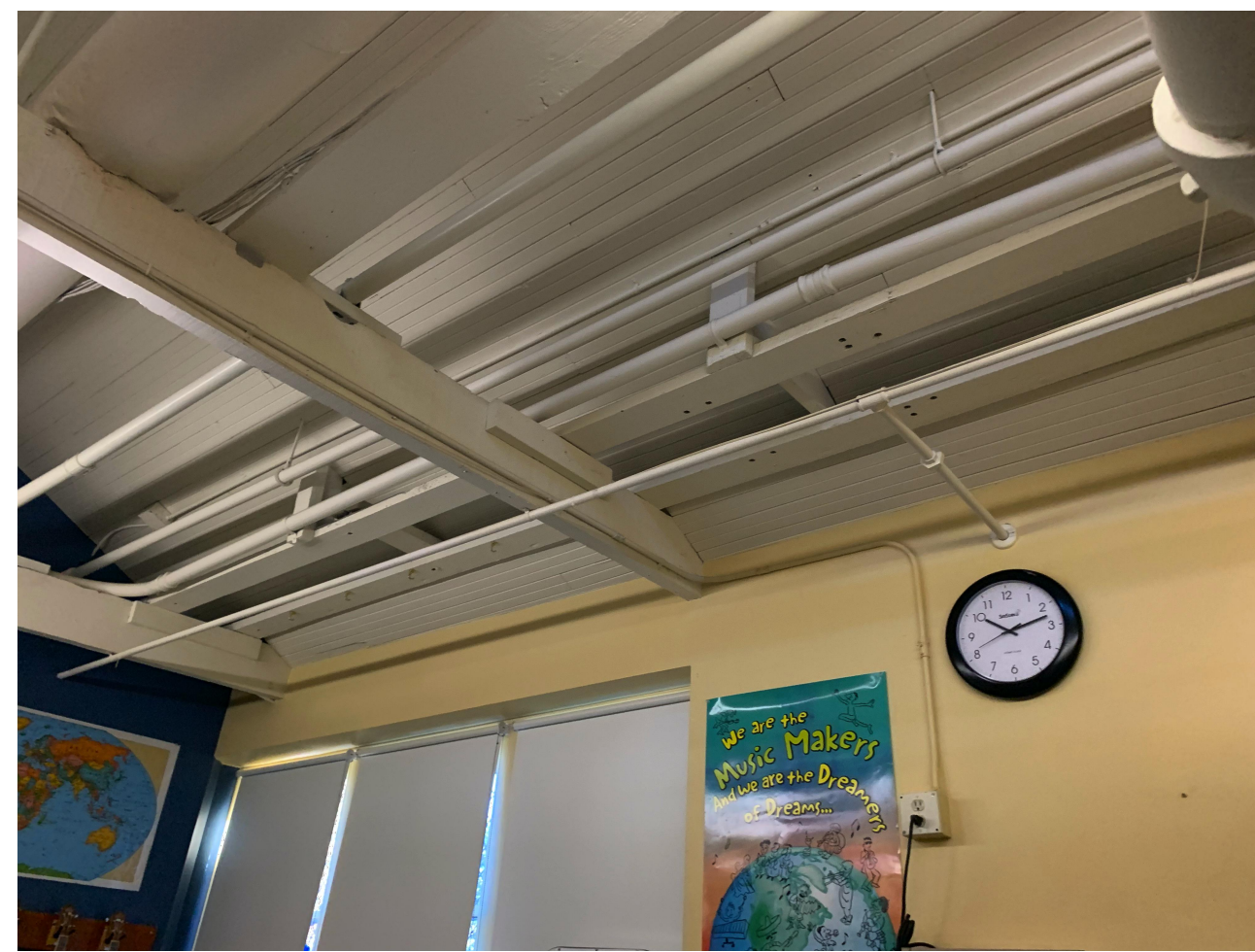
6 SOUTH ANNEX CLASSROOM A702
